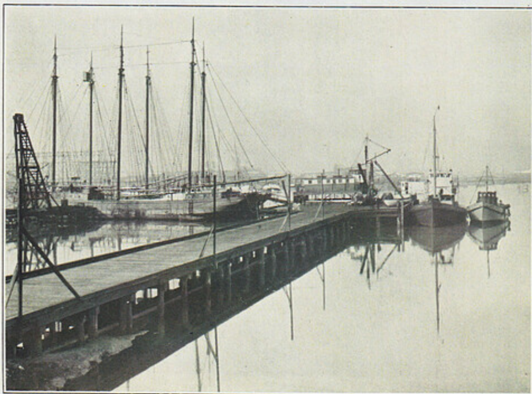
PRIVATE DOCK SHOWING BOATS IN WHICH ATLAS-IMPERIAL ENGINES ARE BEING INSTALLED.
